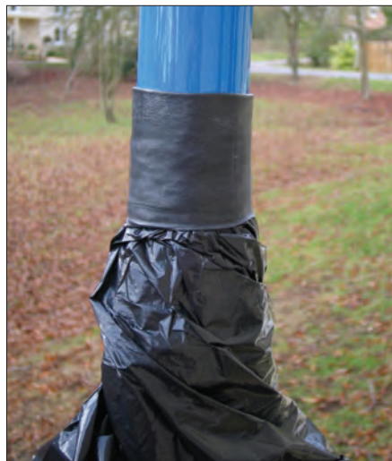
Fig. 4: A short length of the bicycle inner tube is first rolled on to the fibreglass tube and then left in position until it becomes necessary to protect the coupler etc. from rain (see text).
